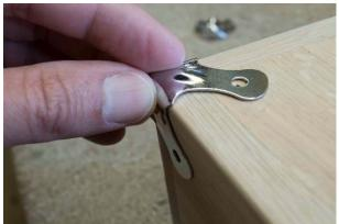
**11)** Check round over with corner hardware. An initial pilot hole has been drilled in the top for the corners. You will have to drill the remaining holes for each of the corners provided. Now is a good time to drill these remaining screw holes.
